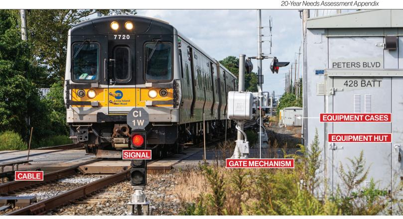
Above, standard LIRR signals system annotated with signals components
