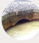
Culverts Are designed to allow water to flow underneath tracks to manage drainage and prevent flooding.
