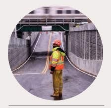
Undergrade bridges Allow an obstacle to pass under the railroad (i.e., the track(s) are on the bridge structure).
