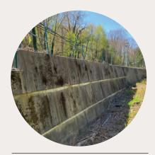
**Retaining walls** Built to hold back soil and provide or keep steeply sloped surfaces track bed.
