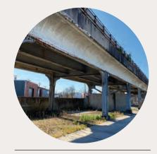
Viaducts Provide separation of the railroad from the surrounding community or allow our rail system to traverse a wide valley with a bridge-like structure.
